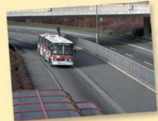
The Ontario Transitway, Ottawa, Ontario
