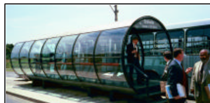
Simple design provides shelter and a raised platform on a limited budget -- Curitiba
