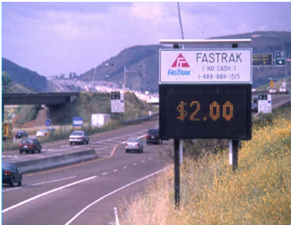
San Diego HOT lane varies the toll through the day and night to ensure free-flow travel at all hours.
