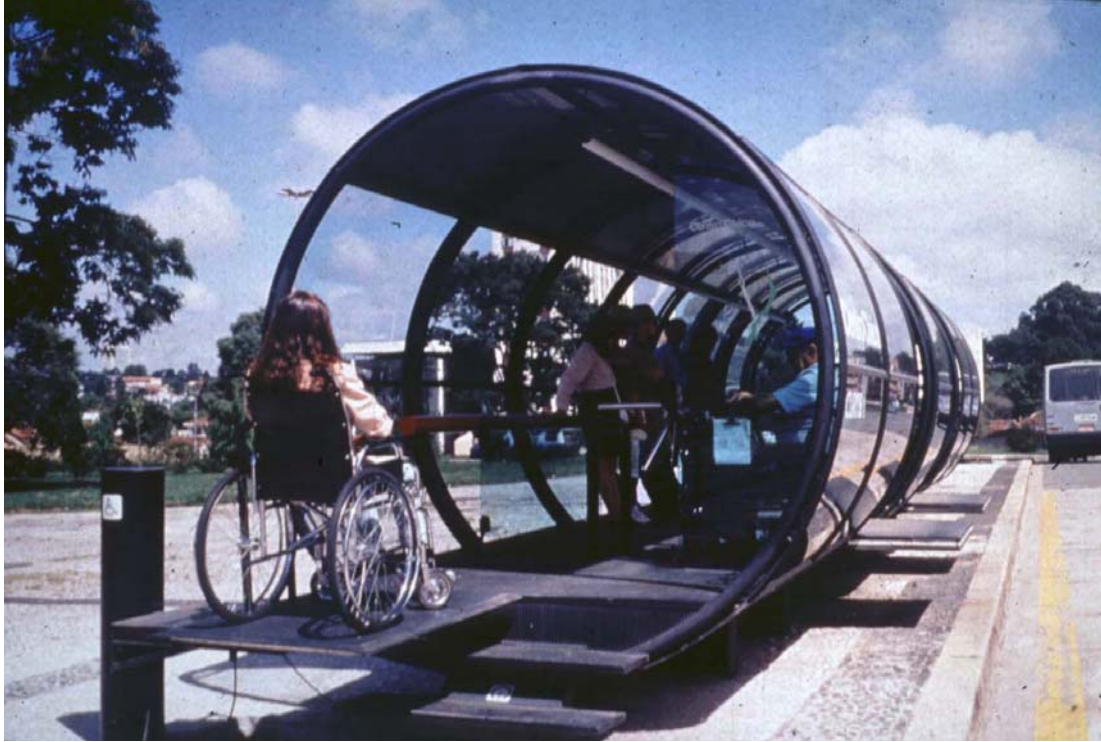
Neighborhood station with wheelchair lift
